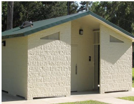
Exterior split block reveal and metal roof, as shown, are optional
